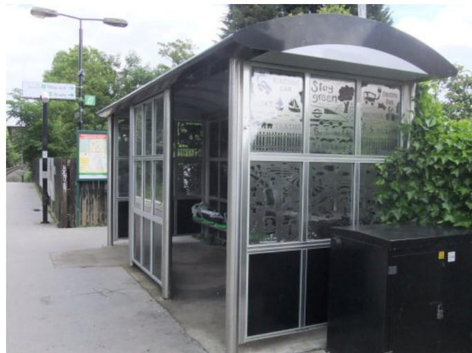
The new vandal-resistant shelter at Garston (above) and one of the laser-cut steel panels (below)
